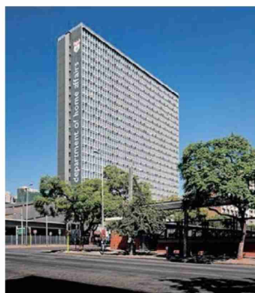
THE Hallmark Building, the head office of the Department of Home Affairs in Pretoria, is one of the buildings with a number of occupational health and safety concerns for workers. | FILE
